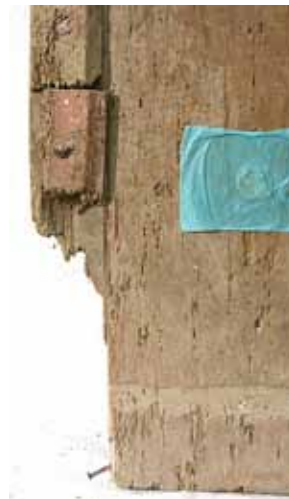
Сл. 7,1. и 7,2. Дрвени додавки Fig. 7, 1 and 7, 2 wooden supplements
